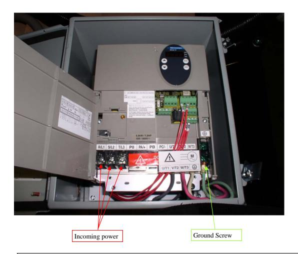
Connect incoming power to the smaller enclosure, it houses the variable frequency drive.
